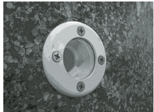
Return faceplate installed.
